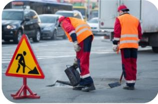
2. Apply Durapave Emulsis RS1 tack coat for enhancing adhesion.
