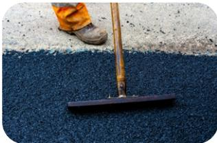
3. Fill the pothole with ready-mix 30 mm above the existing surface and carry out compaction
