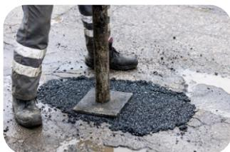
4. The periphery of the patch should be compacted first. To prevent initial inwards pick up of the loose mix, continue to wet the hand rammer with water or place empty plastic lined bags on the loose mix.
