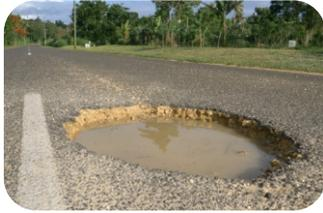
1. Pothole should be cleaned with a stiff wire brush and all loose material including dust should be removed with a soft brush.
